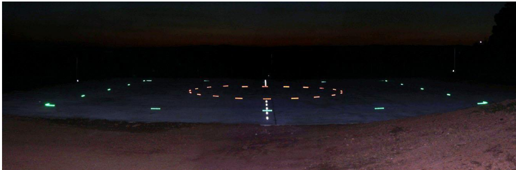
Figure 6: Effect of lighting with LED strip lights for the TLOF, TDPM and FTAG
