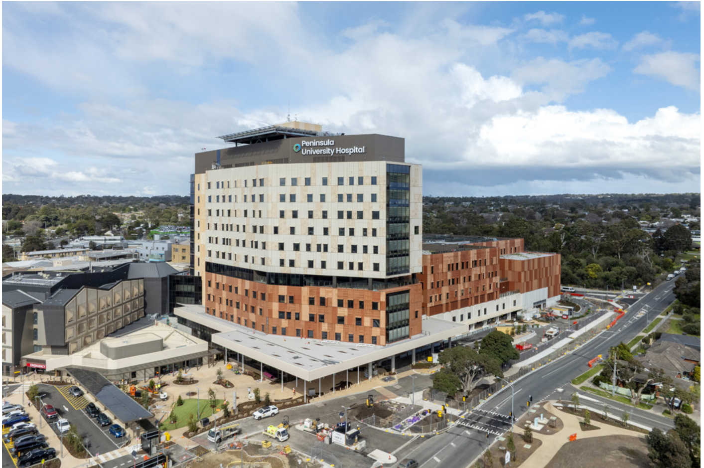
Image 3: Frankston Hospital Redevelopment
