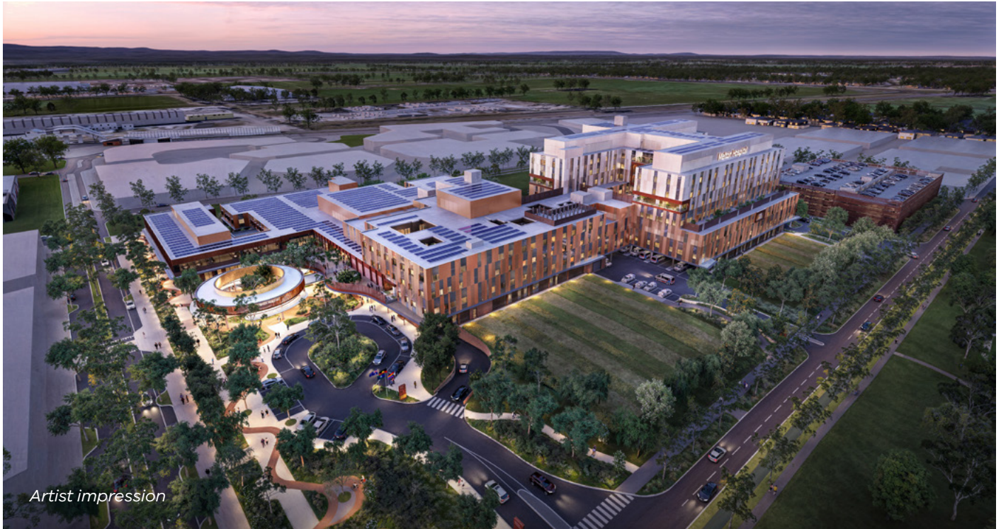
Image 1: New Melton Hospital
